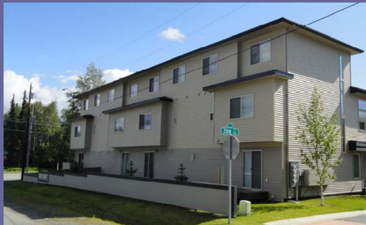
Rear Façade on side street
