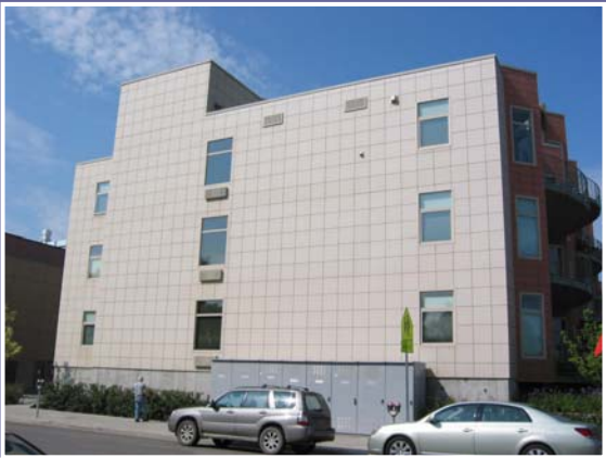
Cordova Street Facade
