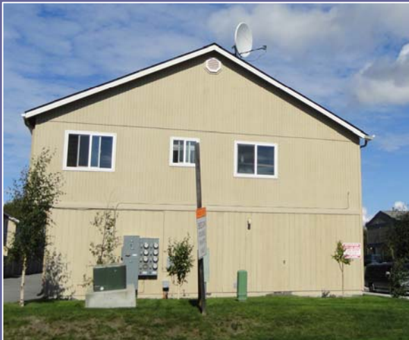
End Façade on side street
