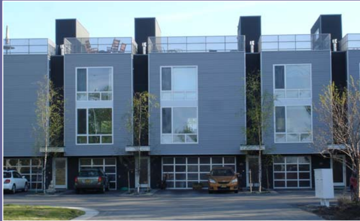
Front Entry Facade
