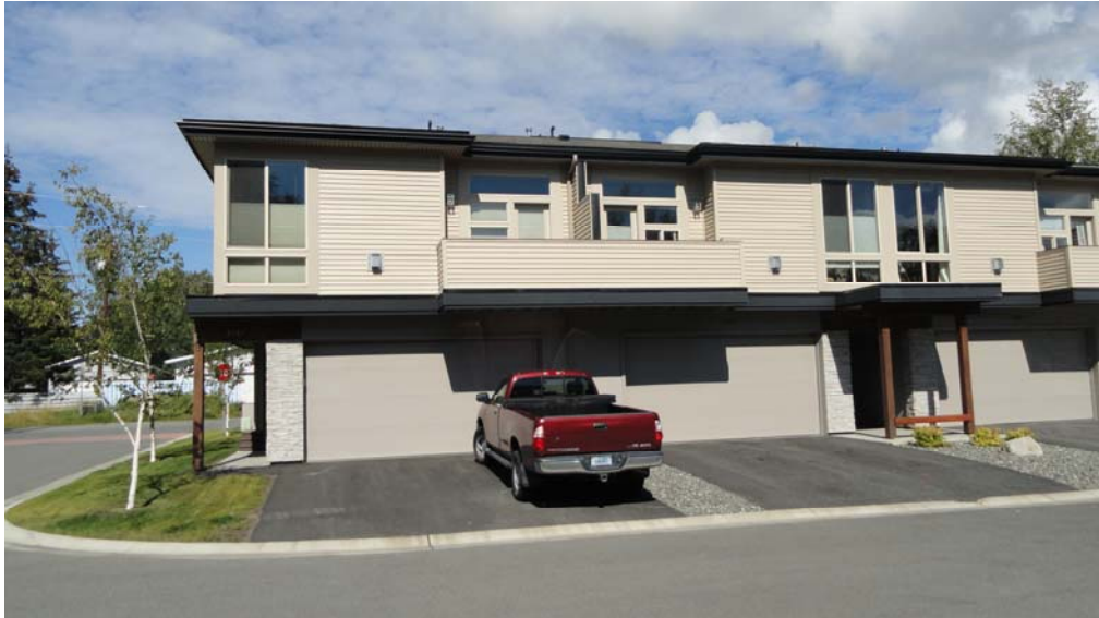
Front side of Units 16 and 17, in four-unit structure on Zion Court (2014)
