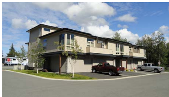
Zion Court units 16 – 19 (Municipality of Anchorage, 2014)
