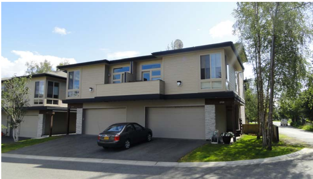
Front of Units 1 and 2, in two-dwelling structure at corner of O'Brien Street (2014)
