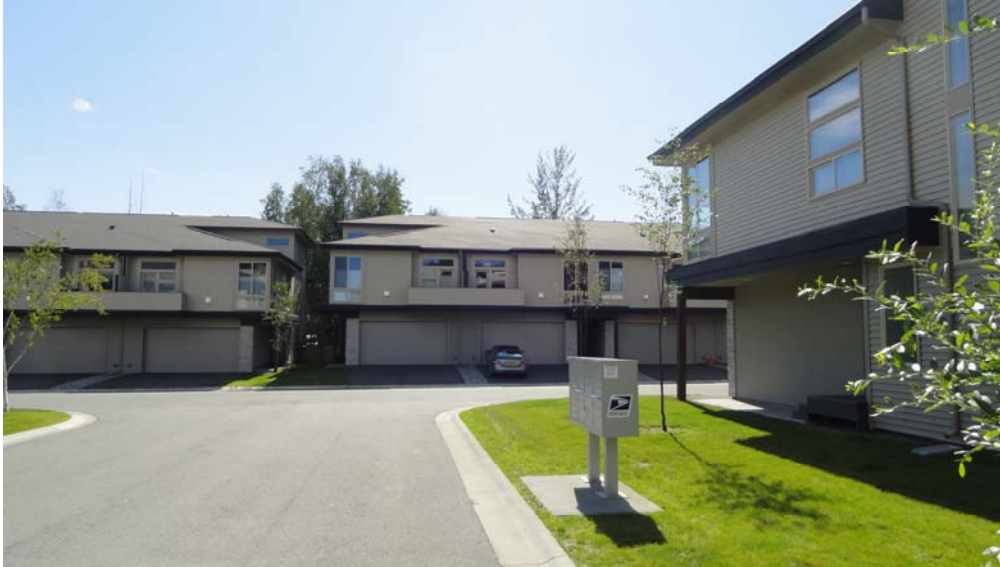
Private street entrance into Zion Court from E. 74 th (2014)
