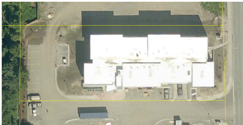
Satellite image of Building A site under construction (Municipality of Anchorage, 2012)
