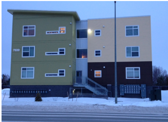
Street-facing Façade of Northwood Apartments Building A (Municipality of Anchorage, 2012)
