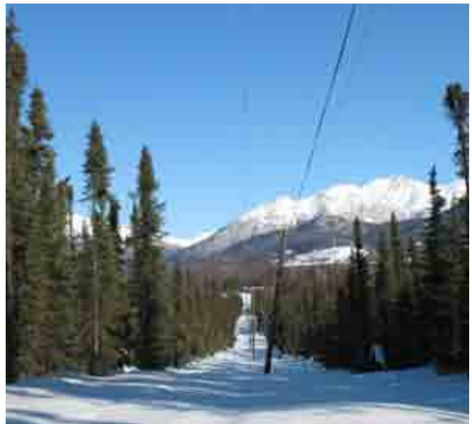
Utilities serve the park but also have scenic impacts and encourage problematic access. As possible, the various lines should be undergrounded.
