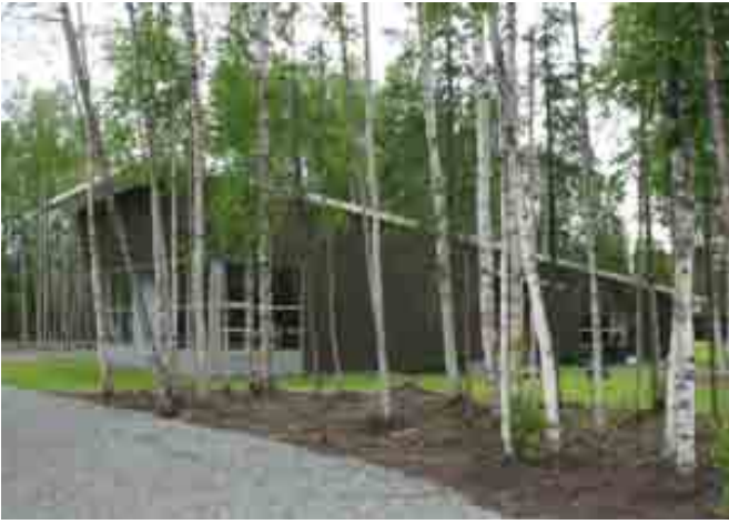
As demand for the park grows and the population of the area substantially expands, existing facilities (such as the ski chalet above), parking, and potentially even multi-use trails may reach capacity and require expansion.
