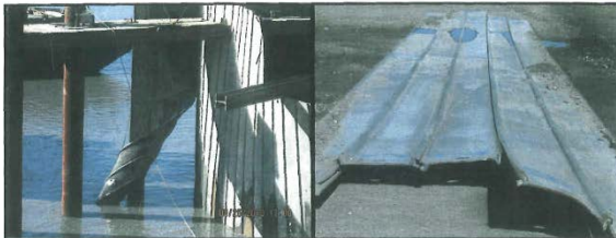
Examples of separated interlocks – WBB Cell 36 (left), face sheets pulled from NE Cell 39 (right).
