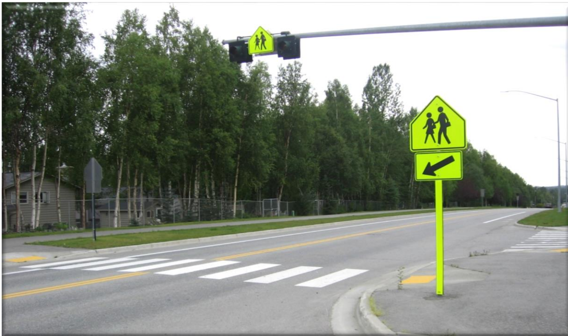
Figure 1. School Crosswalk with Overhead Flashing Beacon and Signing for Scenic Park Elementary
