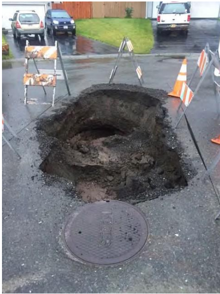
Above left: Sinkhole due to failed pipe on 71 st and Cheryl. Above right: Deteriorated pipe with no bottom on Bennett Street. Lower right: Deteriorated pipe with no bottom on 74 th and Rovenna
