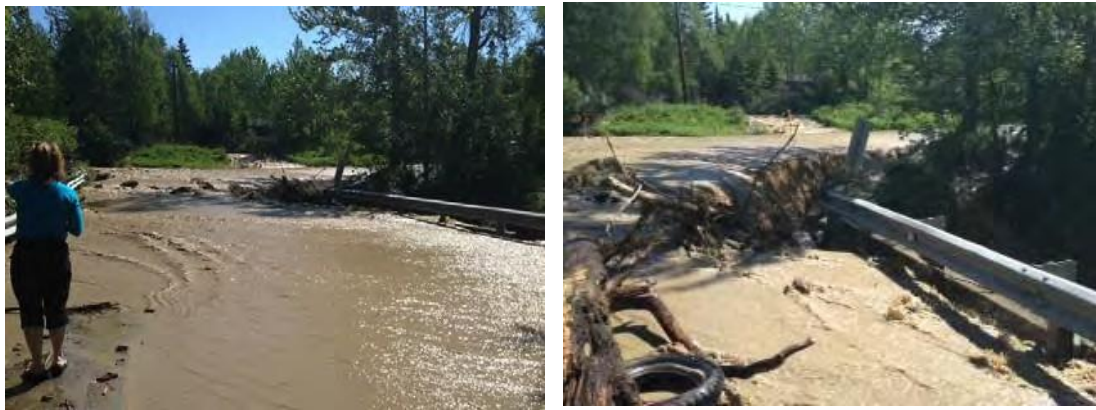
Above: Roadway erosion due to a culvert washout at Porcupine Trail Road. Below: Flooding and damage due to culvert blockage at 140 th and Buffalo Street
