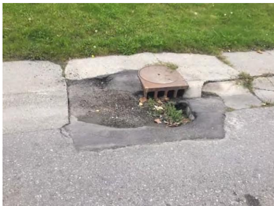
Above: Sinkhole from pipe failure on Prosperity Drive. Right: Sinkhole from pipe failure at Sharon Street.
