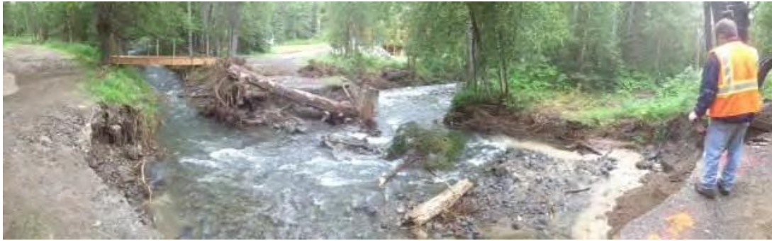
Above: Roadway erosion due to a culvert washout at Porcupine Trail Road. Below: Flooding and damage due to culvert blockage at 140 th and Buffalo Street
