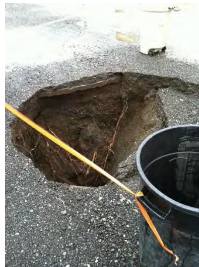
Above: Sinkhole from pipe failure on Prosperity Drive. Right: Sinkhole from pipe failure at Sharon Street.
