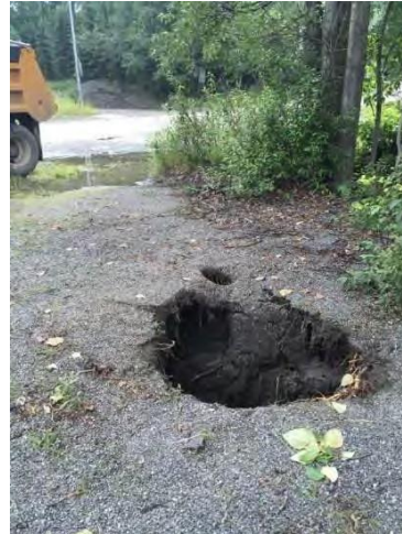
Above left: Sinkhole from pipe failure at Communications Avenue. Above right: Sinkhole from pipe failure at Nichols Street. Lower left: Pipe failure on C Street
