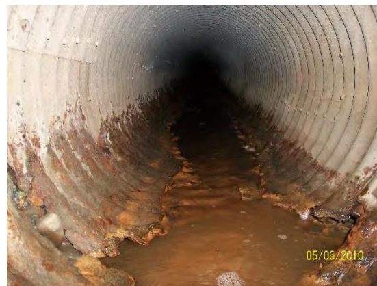
Above left: Sinkhole due to failed pipe on 71 st and Cheryl. Above right: Deteriorated pipe with no bottom on Bennett Street. Lower right: Deteriorated pipe with no bottom on 74 th and Rovenna
