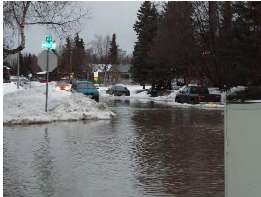
Above: Sinkhole due to failed pipe on North Park Drive. Right: Deteriorated structure with no bottom at 7 th and C St. Below: Flooding from icing on Chester Creek at Arctic Blvd.
