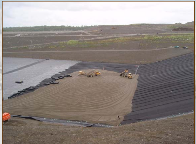
Cell construction showing liner, cushioning fabric and gravel leachate conveyance layer
