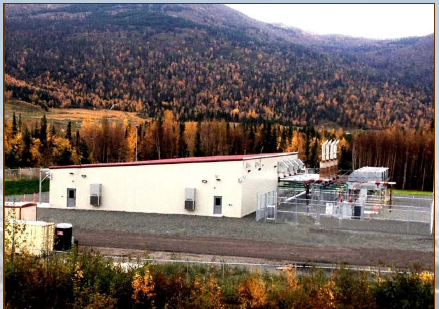
Doyon Utilities Landfill Gas Power Plant
