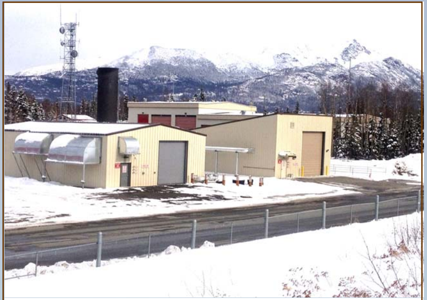
Gas Processing Facility with original blower building adjacent and enclosed flare in background
